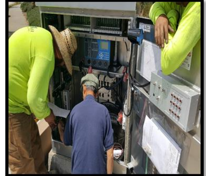
Installation of New Cabinet
